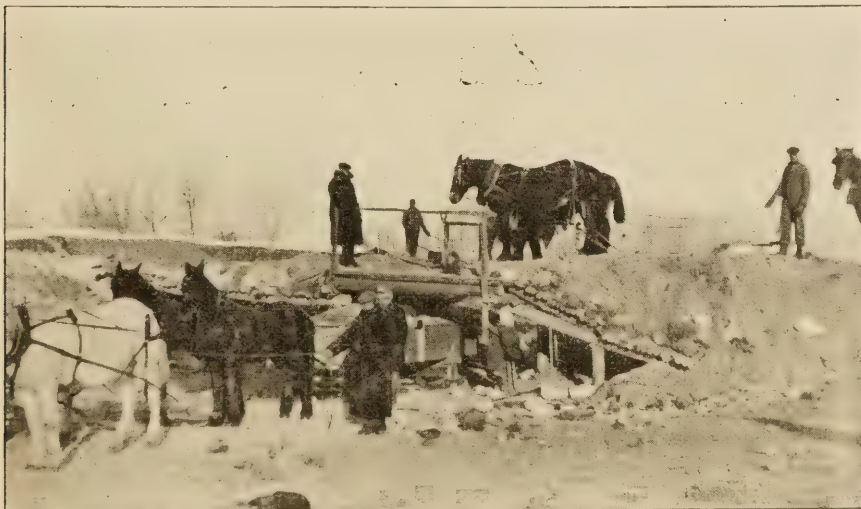
WINTER ROAD WORK IN MINNESOTA. LOADING SLEIGHS BY TRAPS ON MARSHALL COUNTY PROJECT.
